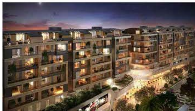
KORU FLORYA RESIDENTIAL COMPLEX AND SHOPPING MALL
